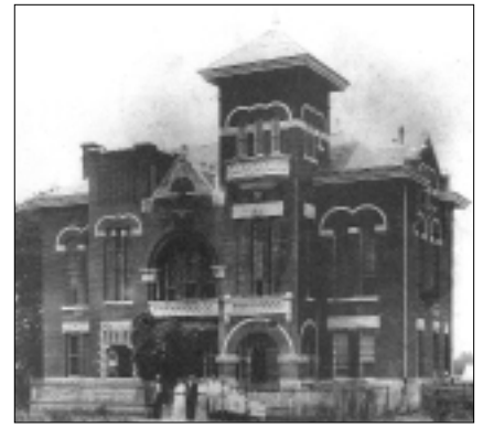
The Fort Bend County Jail housed a gallows on its third floor.
