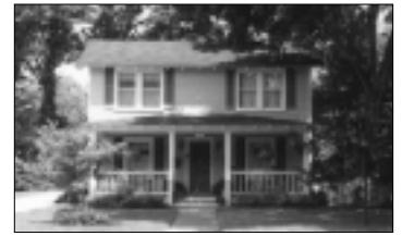
This 1920 I-House is located at 704 Main.
