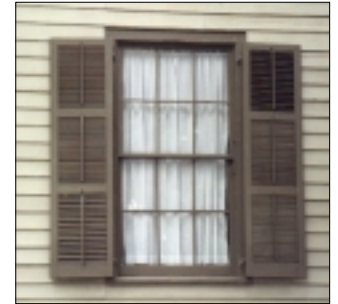
Always preserve historic windows and their original components.
