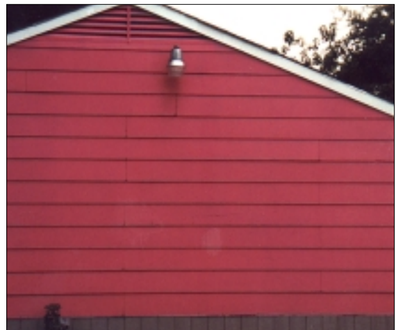
The above example demonstrates the inappropriate use of both synthetic siding and undesirable color choice for the exterior of a building.
