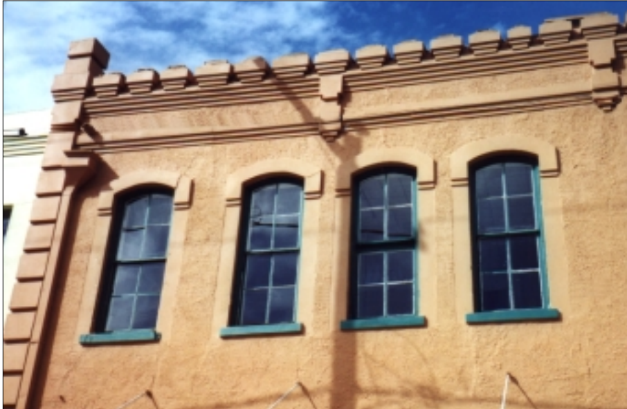
Upper story windows feature a vertical, multi-paned design, providing a visual rhythm across the building and a unity to the streetscape.
