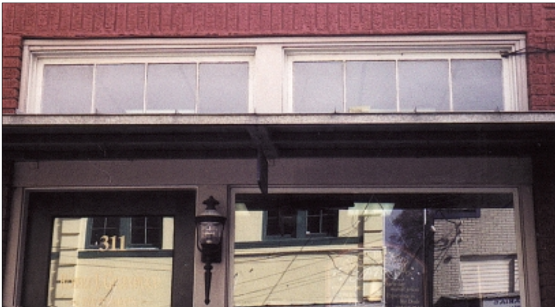
Transom windows lend unity across store fronts, providing both ventilation and light.
