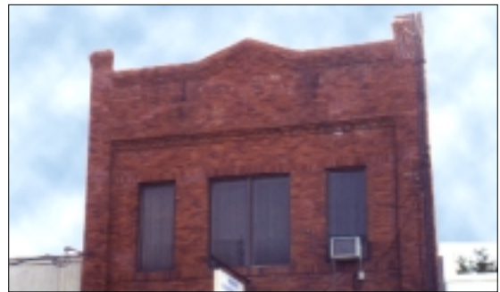
A well-preserved cornice and parapet add to the building's historic integrity.
