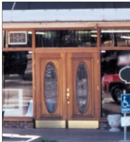
Replacement doors should not attempt to appear historic by the use of stained or etched glass.
