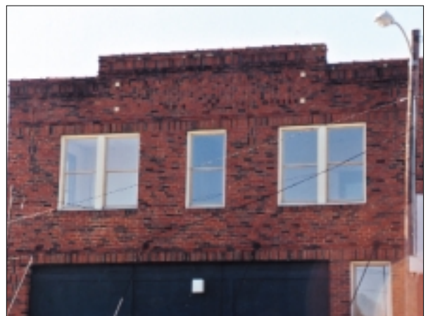
Existing upper story windows should never be replaced with aluminum windows, painted over, or filled in with any material.
