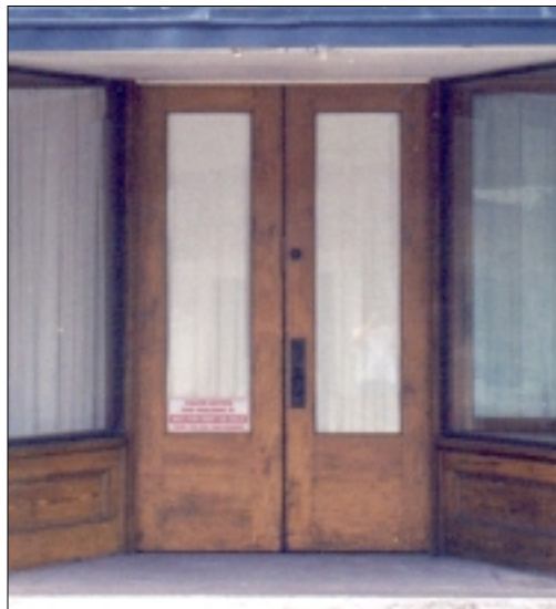
Original door structures should always be preserved whenever possible.
