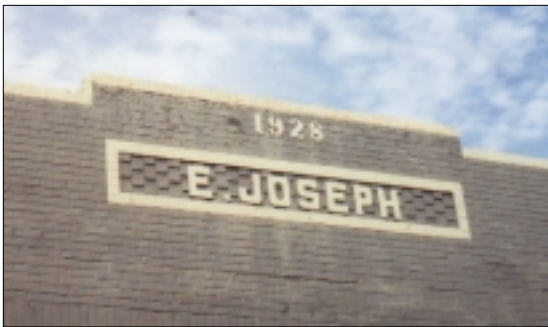
Many parapets contain architectural details, adding interest to the building.
